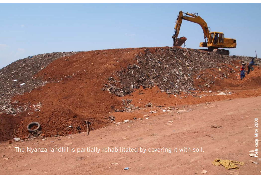
The rehabilitation process involving compaction of the solid waste and covering it with soil after completion in 2011.
