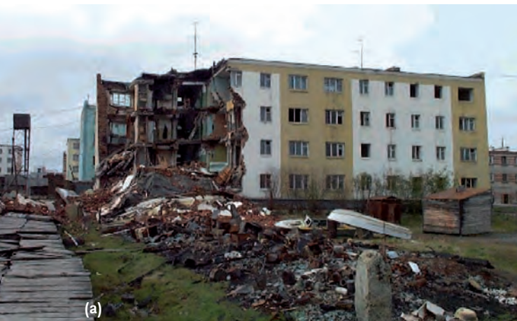
Figure 7.6: Effects of thawing permafrost on infrastructure.
